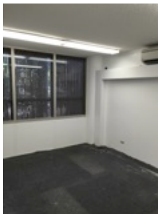
DOUG’S NEW OFFICE SPACE IN PROGRESS
